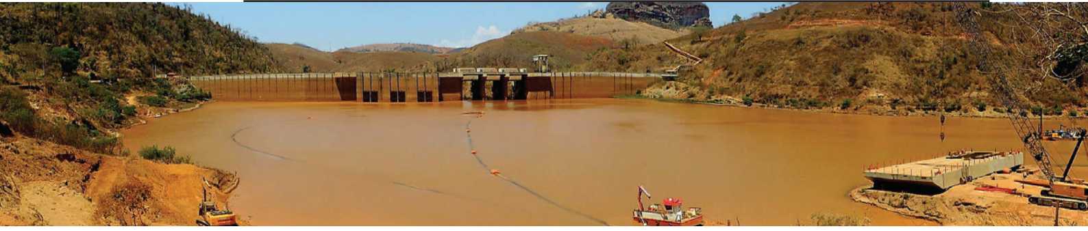
Candonga Dam viewed from upstream (September 2017). The water is visibly loaded with fine sediments. Dredging works were underway.
