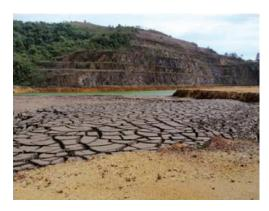
**Figure 4.** Open pit flooded with acid water and used as temporary site for the sludge disposal.
